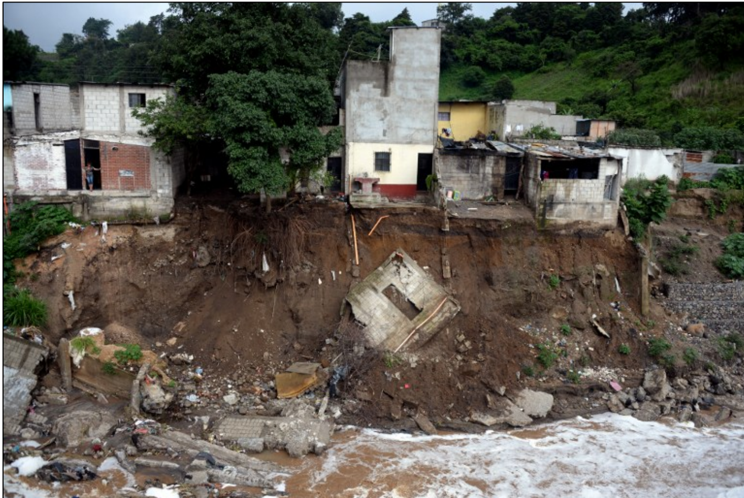
Figure 7. Flood damage associated with Boris near the town of Villa Hermosa, Guatemala, located about 12 miles (20 km) south of Guatemala City. Photo courtesy of Agence France-Presse (AFP).
