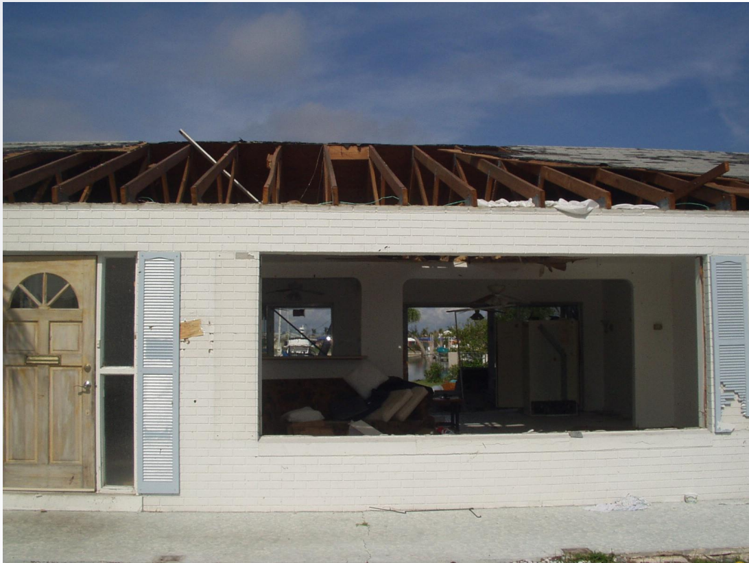
Home built in 1961 (pre-Florida building codes)
