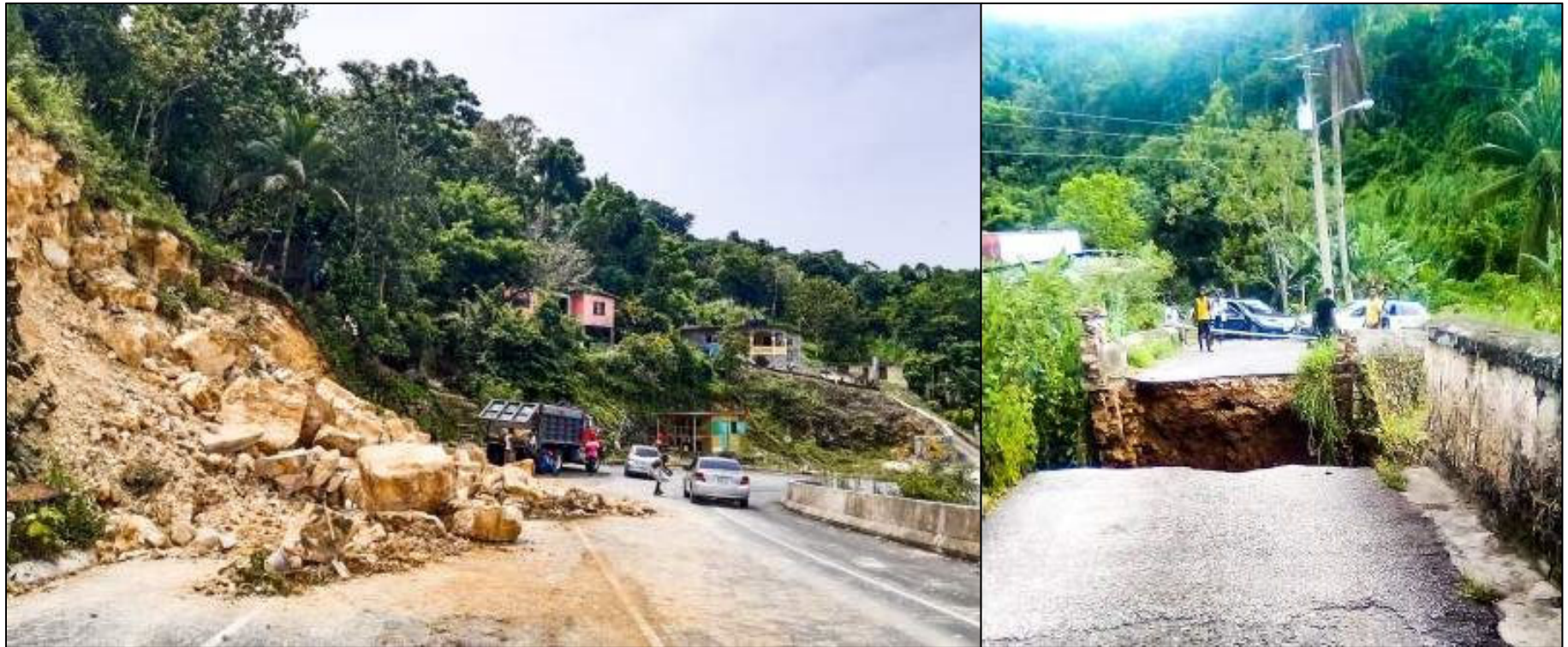
Figure 13. Damage on Jamaica caused by Grace. Left: Landslide debris blocking a road in Westmoreland Parish. Right: Troy Bridge collapse at the border of Manchester and Trelawny Parishes. Photo credit: Jamaica Observer .
