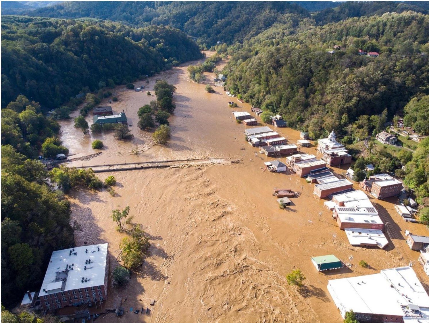
Figure 33. Flooding in Downtown Marshall, NC from the French Broad River after Helene. Photo courtesy of Old Marshall Jail Hotel, taken from the North Carolina State Climate Office.
