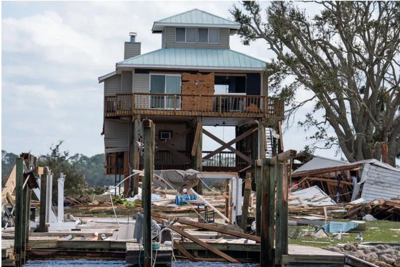
Figure 26. A home in Keaton Beach, FL was gutted due to Helene's 12–16 ft storm surge there. The majority of homes in Keaton Beach were either gutted or washed away. Photo courtesy of Alicia Devine and the Tallahassee Democrat.
