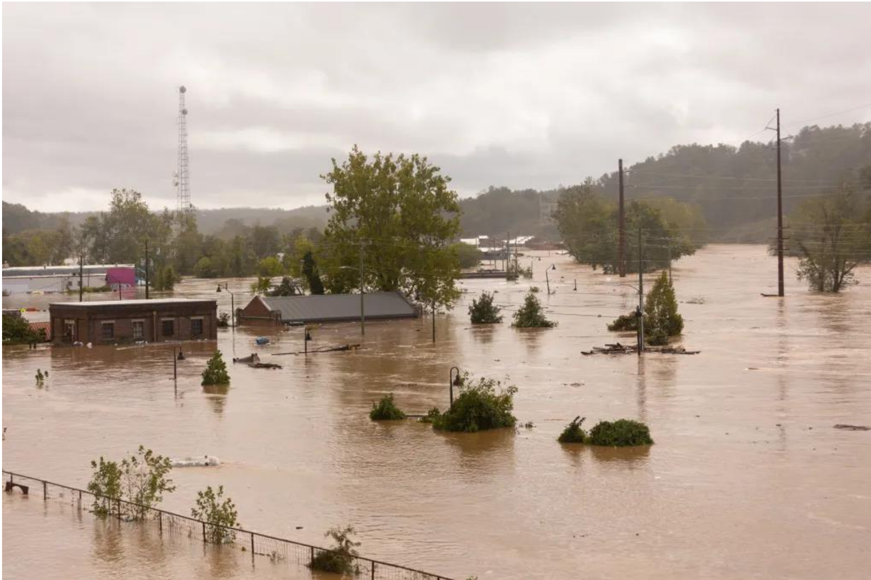
Figure 30. Catastrophic flooding from the French Broad River in Asheville's River Arts District in the aftermath of Helene on 27 September 2024. Image courtesy of Colby Rabon and the Carolina Public Press.
