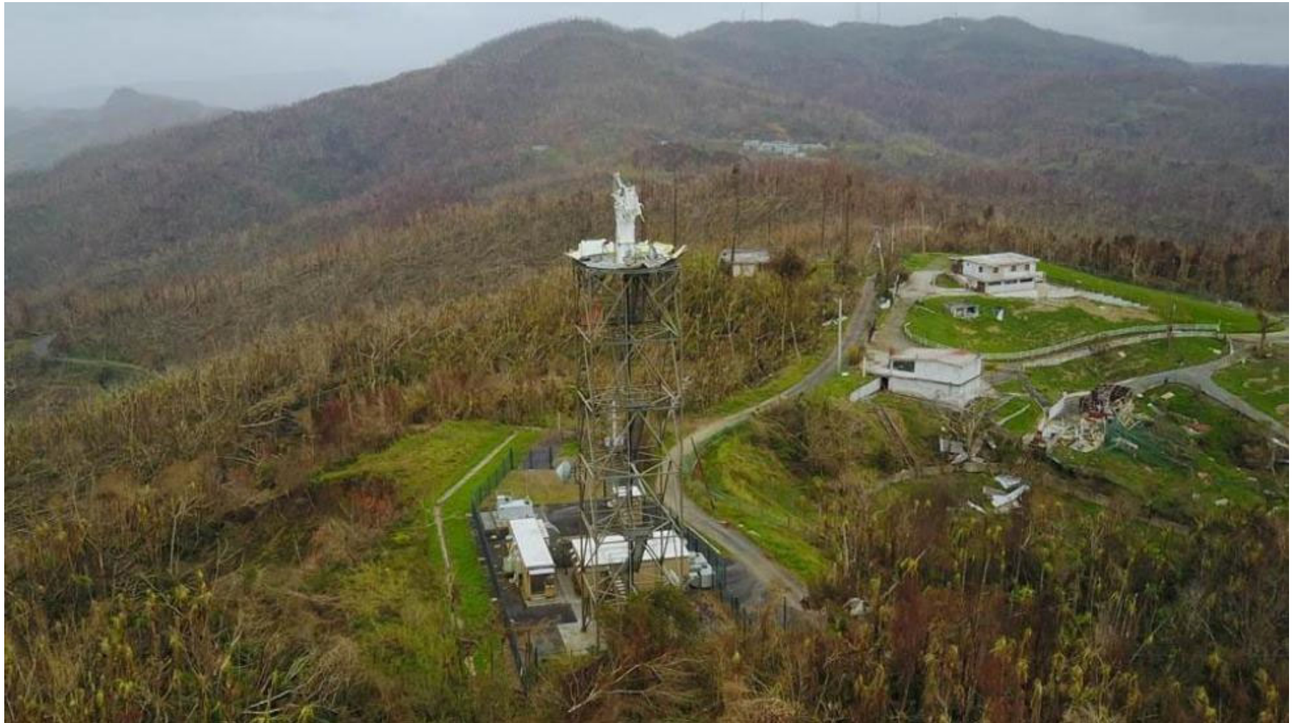
Figure 10. The remnants of the San Juan WSR-88D radar after its destruction by Hurricane Maria. Photo credit: WFO San Juan.
