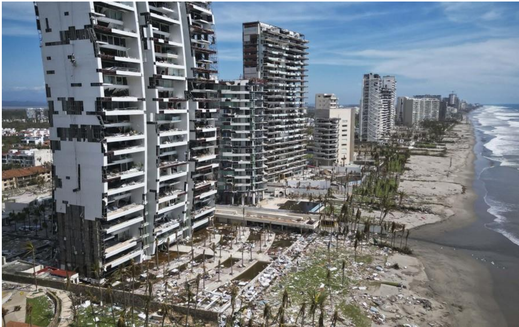
Figure 12. The extreme winds of Otis caused significant damage to high-rise buildings along the coast of Acapulco, Mexico. Photo credit: Rodrigo Oropeza, AFP/Getty Images.
